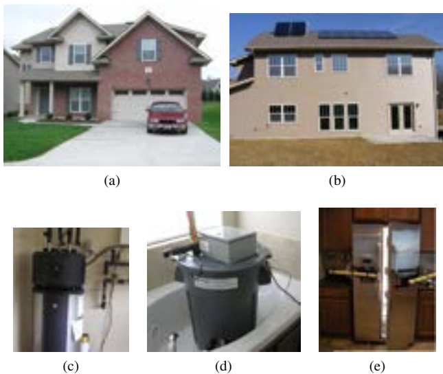
Fig. 1. The near net-zero-energy (NNZE) house front (a) and back (b). TVA robotic devices are controlled to mimic realistic human behavior. Also shown is a HPWH used in the retrofit house (c), a shower emulator (d), and a refrigerator with programmed arms (e) that operate according to automatic schedules.
