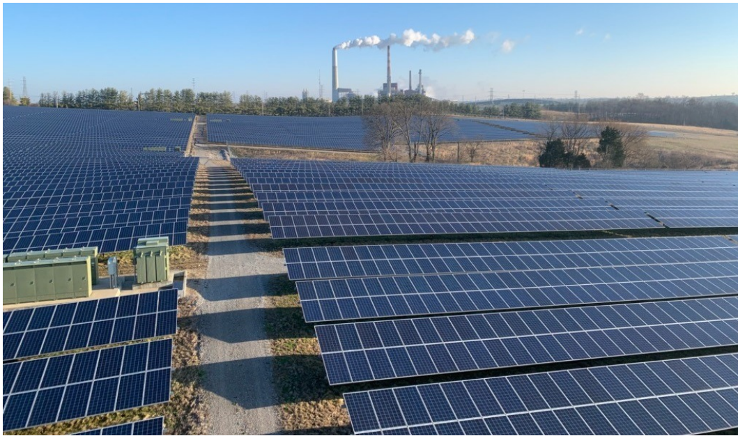
Figure 1. The aerial view of the E.W. Brown generating station, which includes Kentucky's largest solar farm, hydropower plant, natural gas units, and coal fired power plants.
