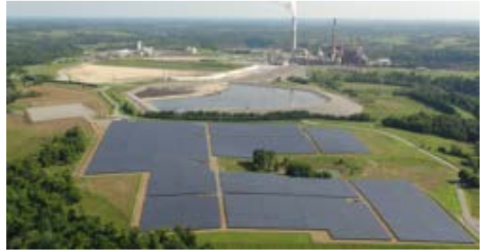
Figure 7. The LG&E and KU E.W. Brown universal solar facility, which houses a 14MW dc 10MW ac PV system. The PV system is divided into ten sections with each rated 1MW ac .
